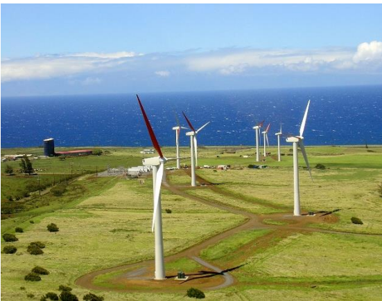
Photo from Hawaiian Electric Light Company, NREL 14697
